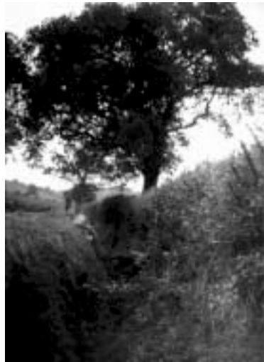
Ditch as seen from road, to show depth, with oak tree in the distance.
